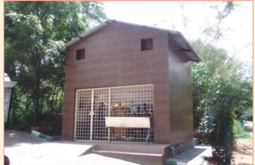
Installation of RO Plant (near chimpanzee enclosure)
