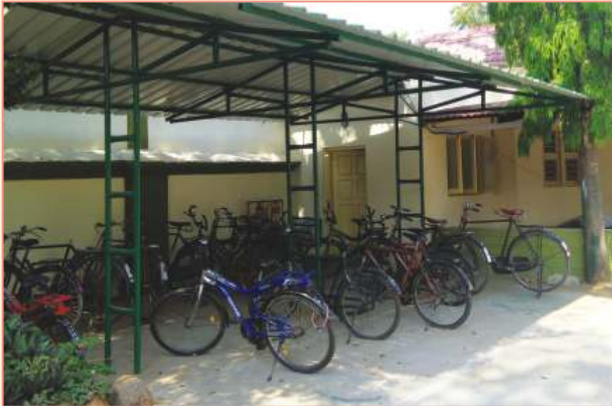
Cycle stands renovation
