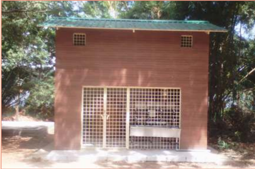
RO plant installation near karanji Boating Point
