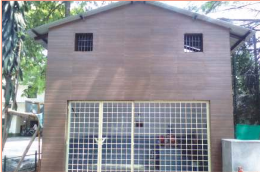
Installation of RO Plant (near food court)
