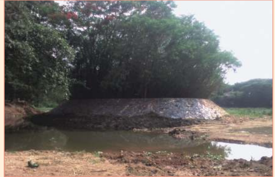
Karanji Island revetment
