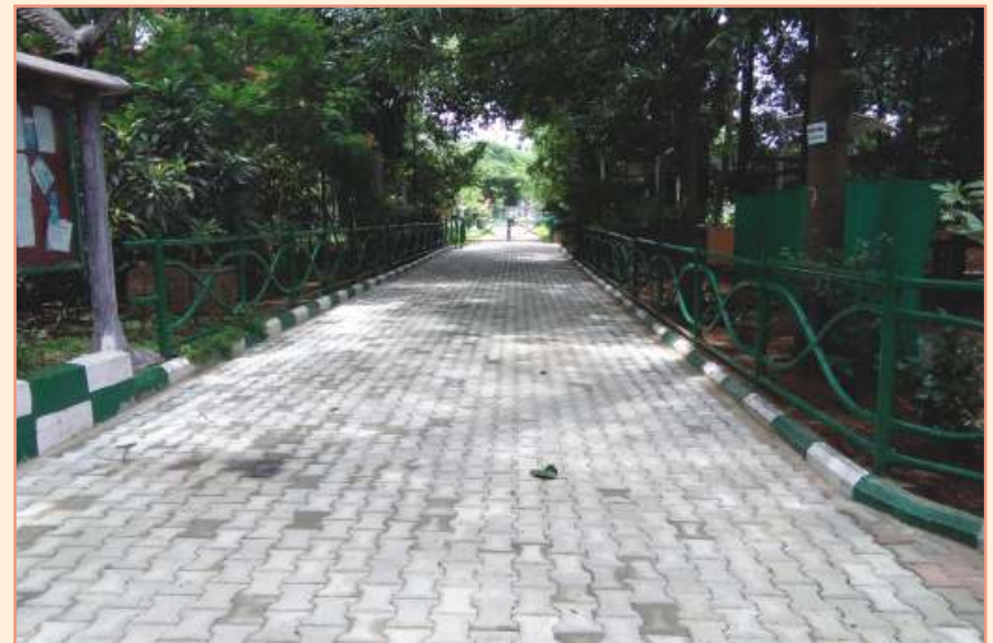
Inter-lock pavement near food court
